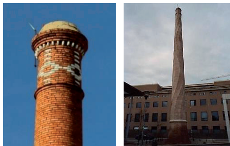
Figure 5: Examples of a decorated crown (left) and stack (right) (right photo from Pallarés et al, 2011)
