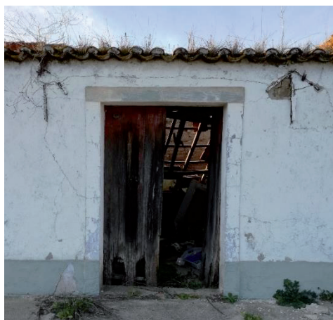
Figure 4: Caramela dwelling detail of iron stabilising rods in Vale da Vila, Pinhal Novo, Palmela, Portugal (2017)
