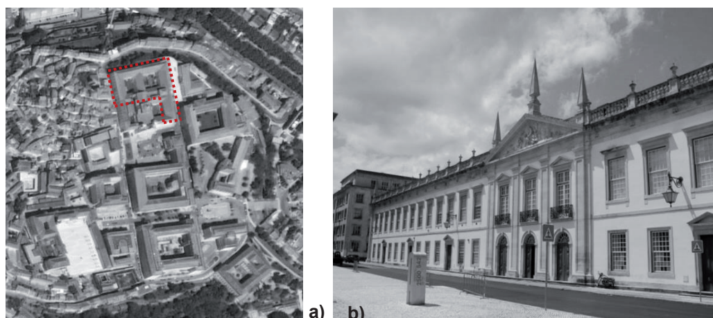
Figure 1: a) Location of the Science Museum of the University of Coimbra (MCUC), [ArcGis (2017)]; b) external view of the Museum East façade
