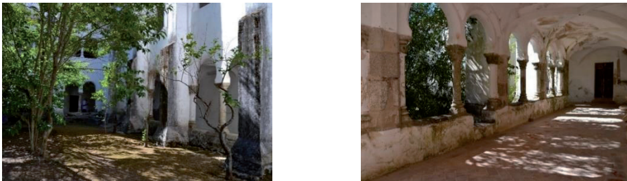
Figure 1: Cistercian atmosphere at Monastery of São Bento de Cástris. Left: Cloister. Right: North gallery of the cloister. Source: Patrícia Faustino, 2016
