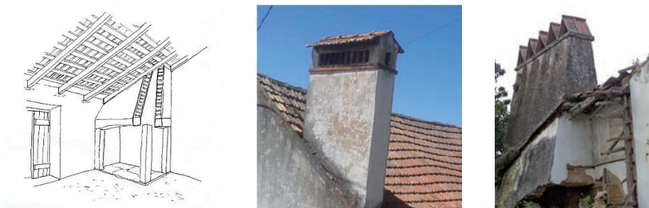
Figure 8: Traditional kitchen and types of smoke canopy
