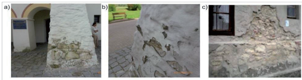
Fig. 15: a, b&c) Opoka walls covered with plaster - historic buildings of Kazimierz Dolny.
