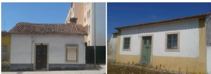
Figure 2: Traditional building typology: a) located in urban areas, b) located in rural areas
