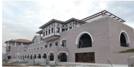
Figure 9: “New” Buildings in Hacı Bayram District. Source: ankara.bel.tr
