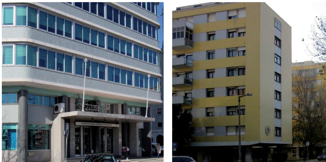
Figure 5: Two buildings with monochromatic flat azulejos in Lisbon. Left: Ministério do Trabalho in Praça de Londres ; right: building at Avenida do Brasil
