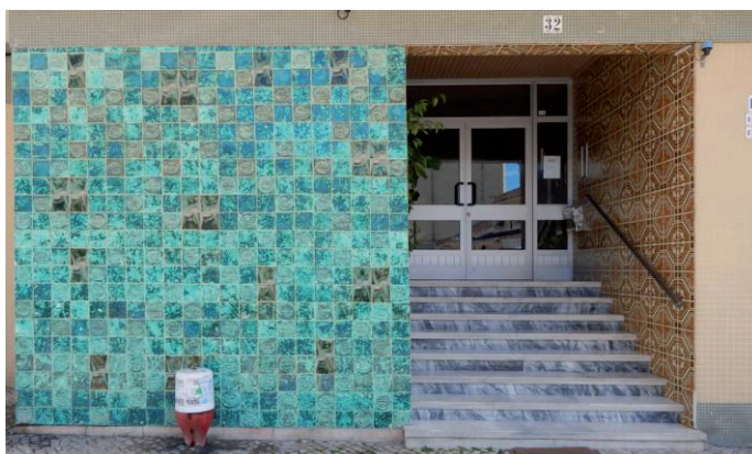
Figure 6: Lining at street level only, with not wholly repetitive pattern. R. Luís Pastor Macedo Nº 32, Lisbon
