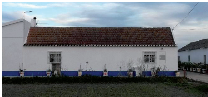
Figure 3: Caramela dwelling located in Lagoa da Palha, Pinhal Novo, Palmela, Portugal (2017)
