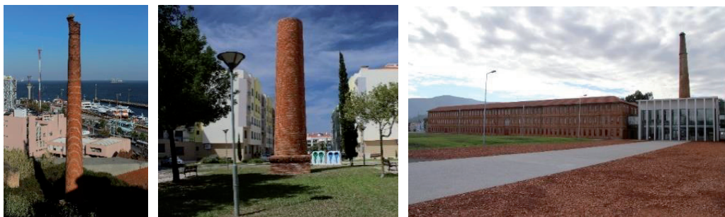
Figure 1: An abandoned chimney in Cacilhas (left). A preserved chimney in the middle of a square in Montijo (center) and the rehabilitated old Arganil ceramics factory (right) (photo from CIM/RC)
