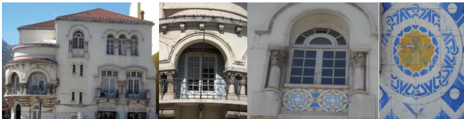
Figure 10: Tiles applied in the facade of the Academic College.
