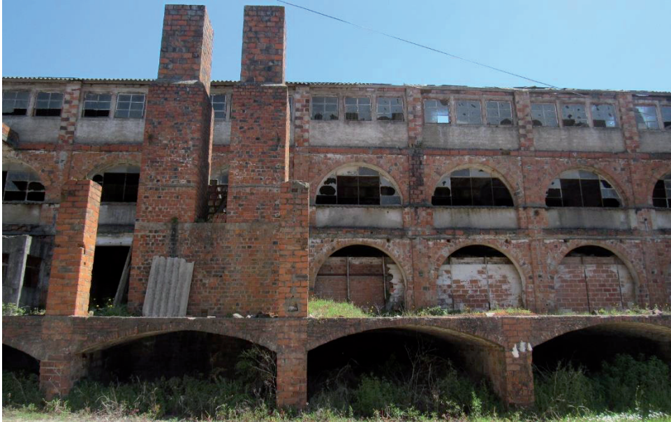
Figure 3: The factory building. Caxarias , 2018
