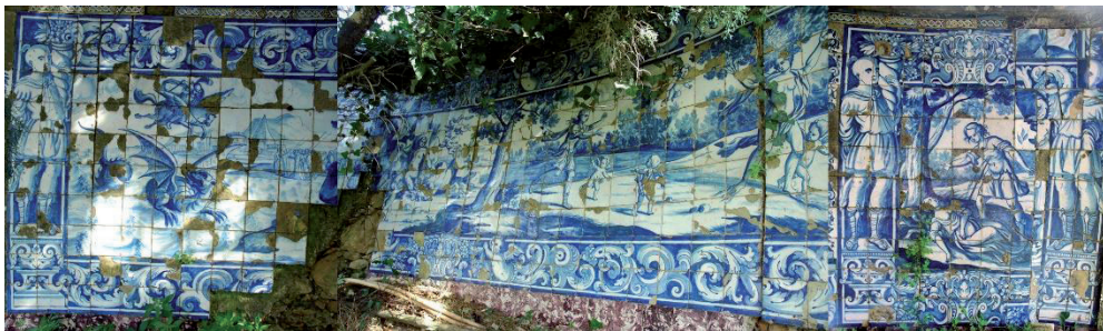
Figure 1: The different scenes of the panel that was still in situ.
