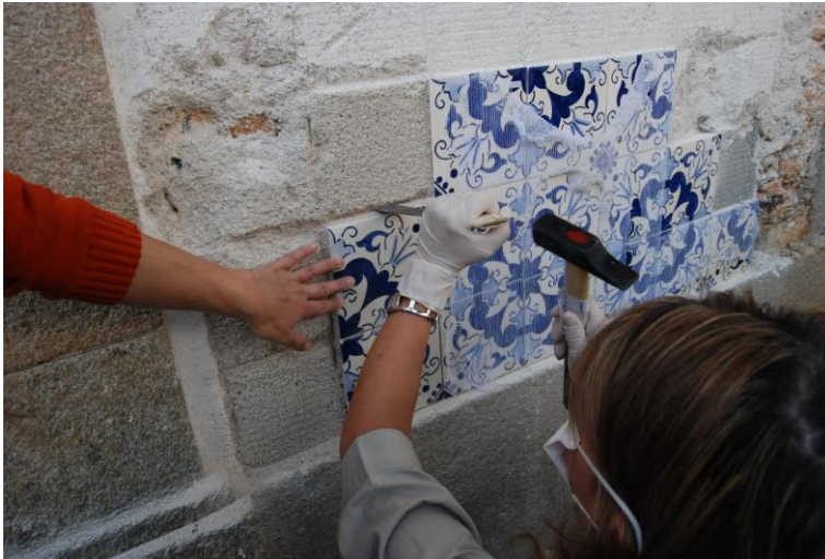
Figure 7 – Removal of mortars based on different binders
