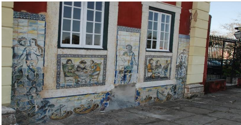
a. NE Turret - Entrance to the Formal Garden.
