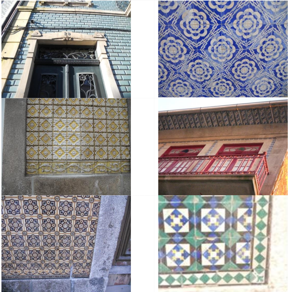
Figure 1 - Variety of patterns in façades
