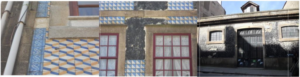
Figure 4 – Typical degradation process
