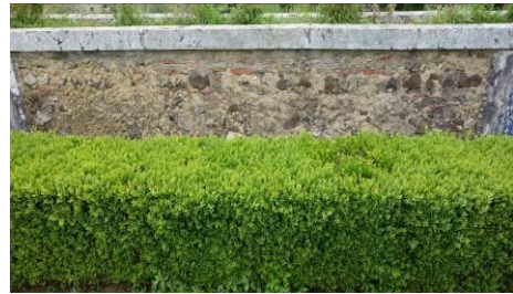
f. Panel removal for conservation.
