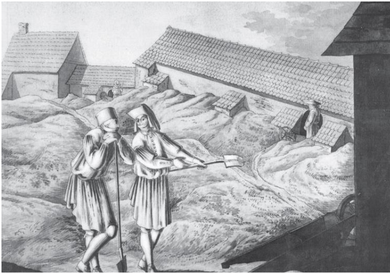
Figure 7. The large amount of accumulated toxic waste (mostly arsenic oxide) that has collected in the smoke chambers is scooped out by workers wearing mouth masks.
